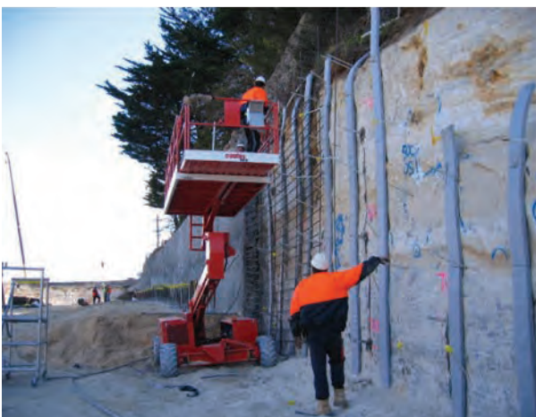
Figure 1: Heavy soil nailing and retaining wall construction for cutting in Banks Wall Sandstone, Blue Mountains, Leura, NSW.
