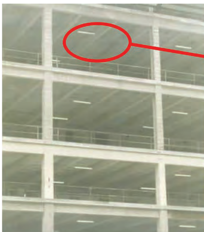
Figure 2: Demountable composite beam
