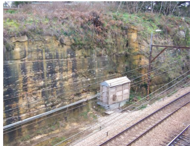
Figure 2: 100 year old unsupported vertical railway cut in Banks Wall Sandstone at Mt Victoria, Blue Mountains, NSW.
